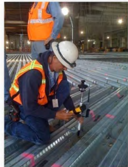
Using Job-Site Solutions, one person can accurately lay out hundreds of points in a single day.
